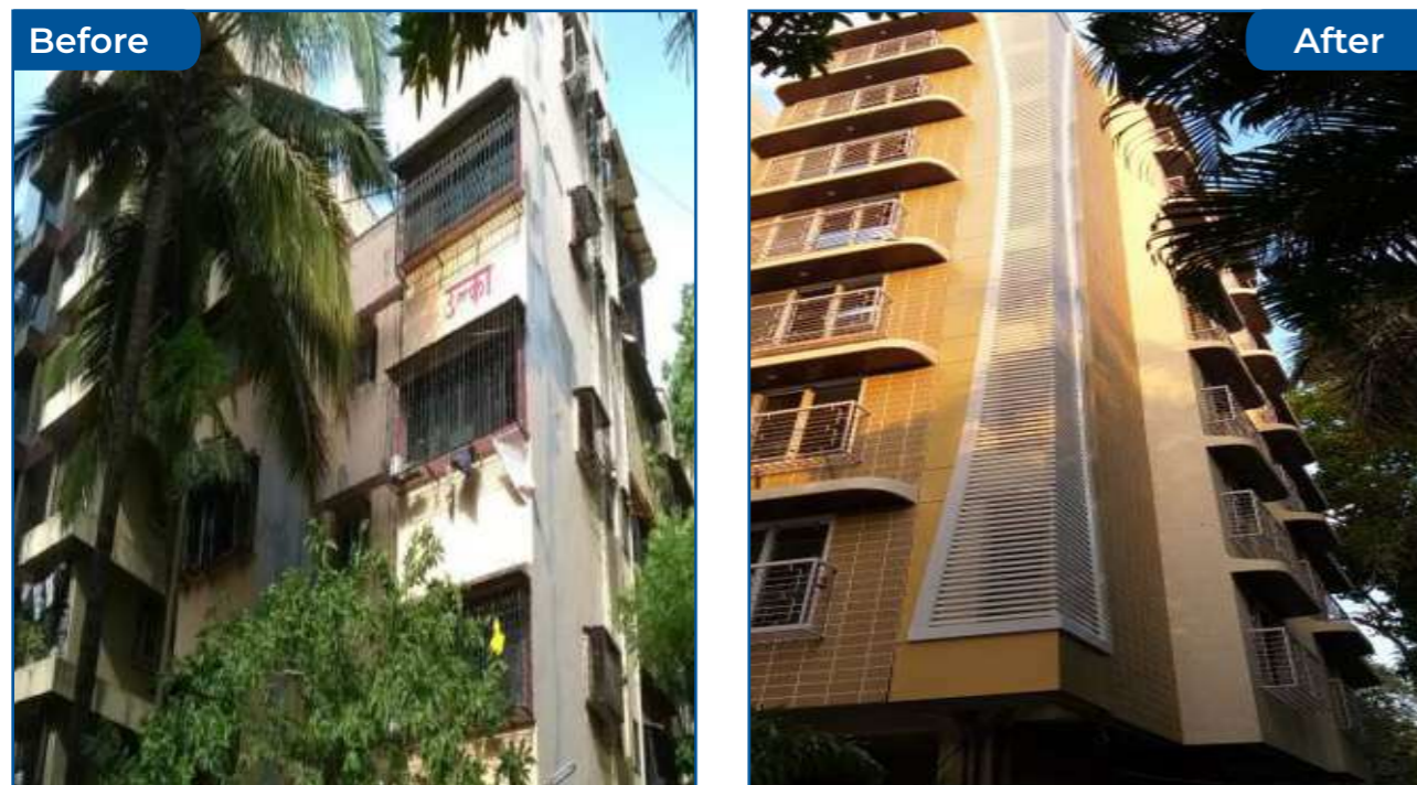
Ulka Co-operative Housing Society Ltd. Borivali (West) | Constructed Area: 27,706.54 sq. ft. | Total Units: 29 | Members Rehoused: 17 Timeline: Completed in 18 months
