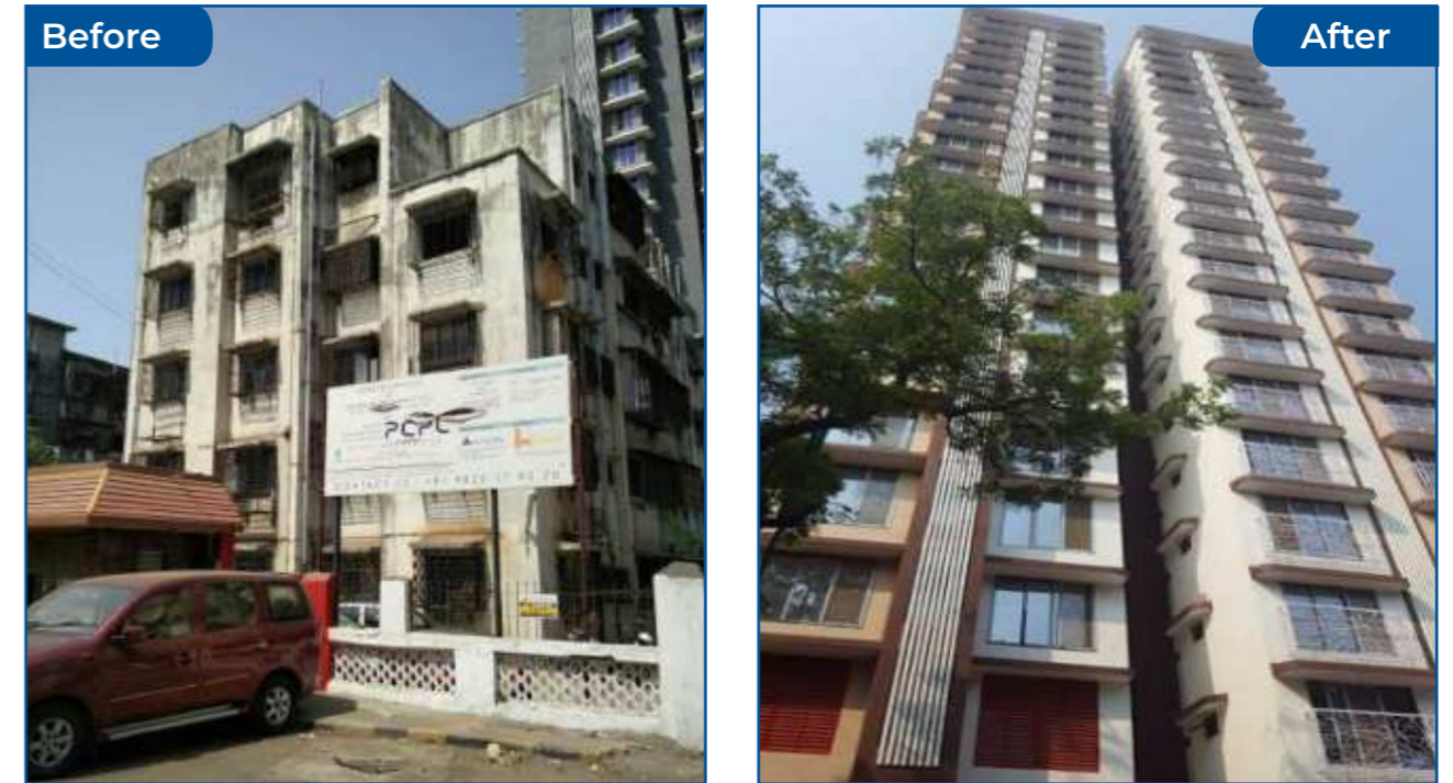
Malad Rajhans Co-operative Housing Society Limited Malad (East) | Constructed Area: 52,380.42 sq. ft. | Total Units: 58 | Members Rehoused: 36 Timeline: Completed in 32 months
