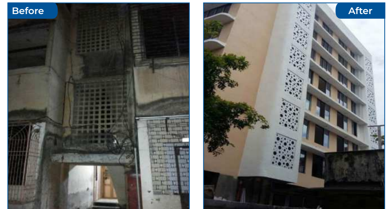
Prachiti Co-operative Housing Society Ltd. Goregaon (West) | Constructed Area: 22,642.94 sq. ft. | Total Units: 28 | Members Rehoused: 12 Timeline: Completed in 16 months
