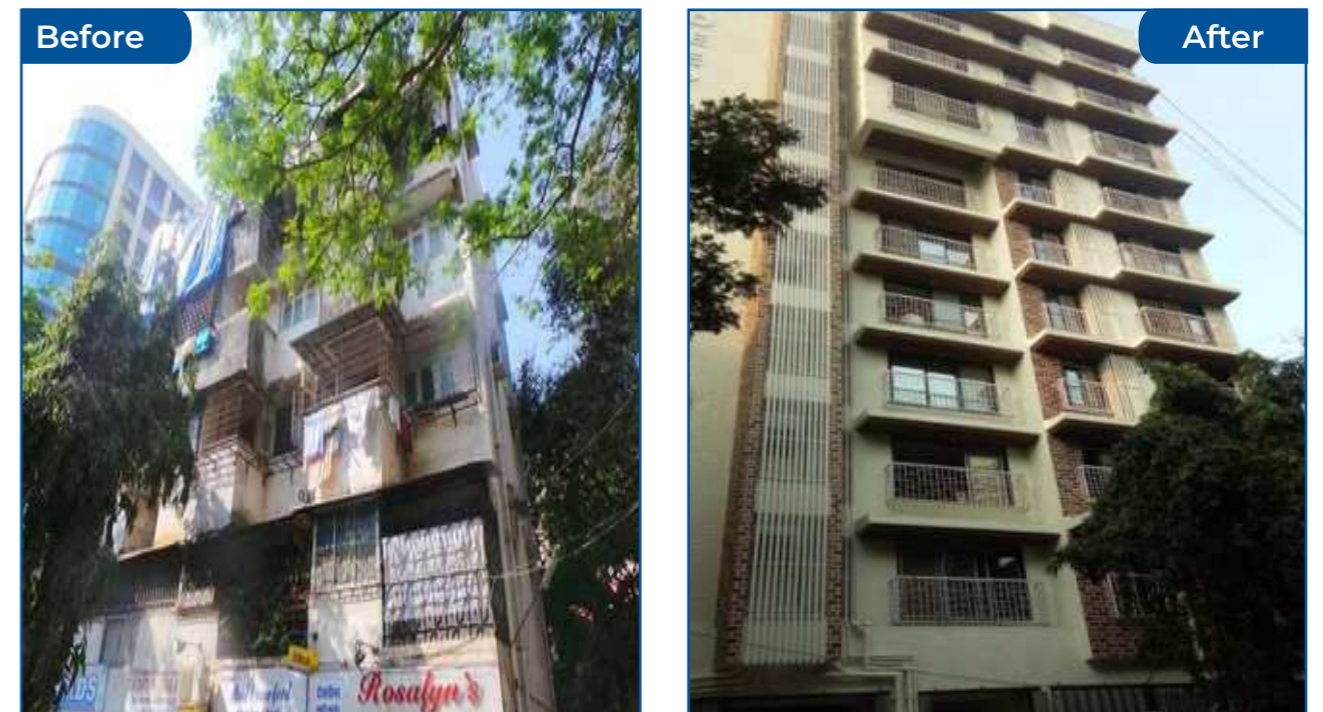
Deep (Sunder Lane) Co-operative Housing Society Limited Malad (West) | Constructed Area: 20,150.21 sq. ft. | Total Units: 31 | Members Rehoused: 22 Timeline: Completed in 26 months
